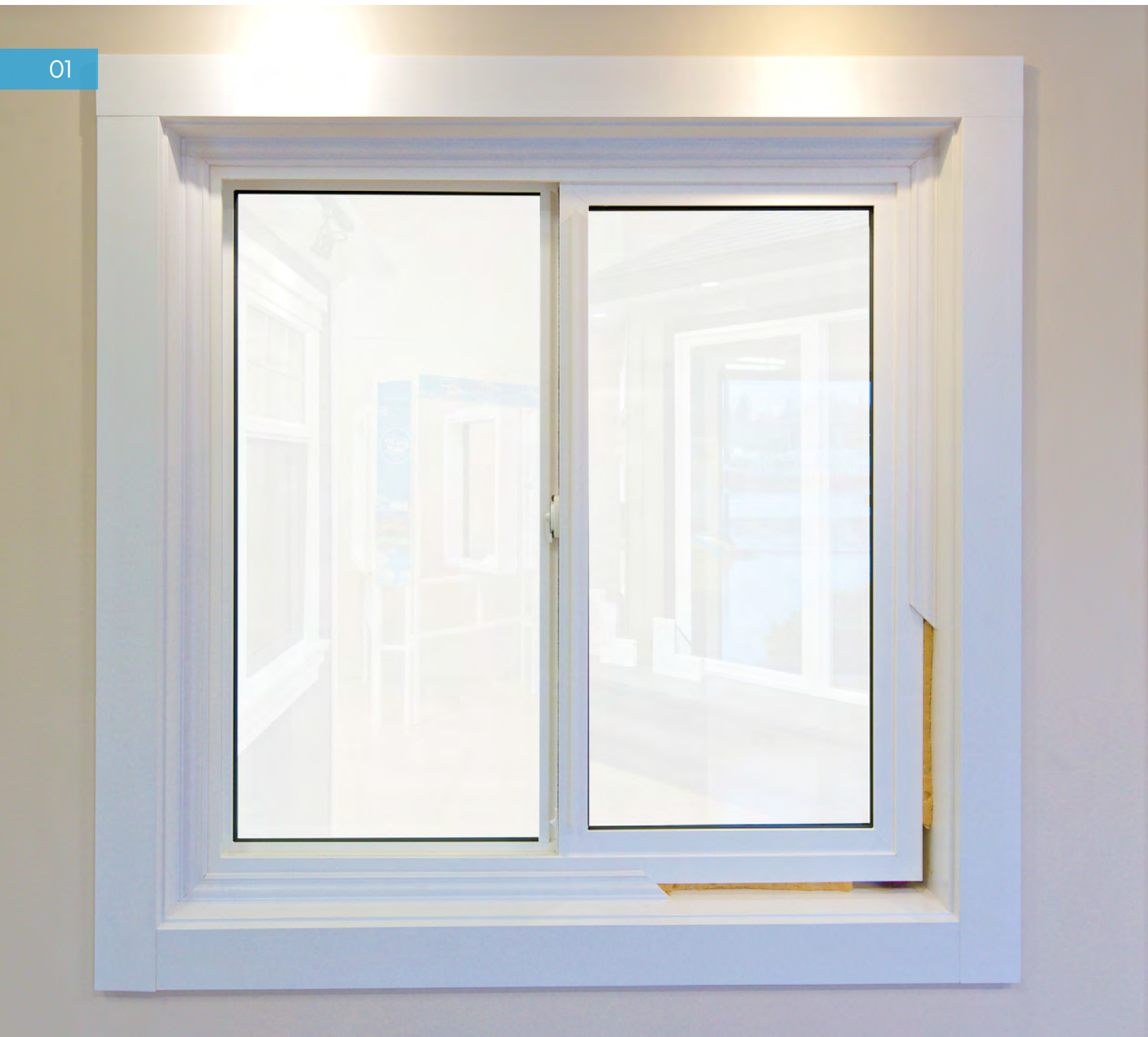
01 DISPLAY WINDOW SHOWING REPLACEMENT INSTALLATION OVER EXISTING ALUMINUM FRAME
